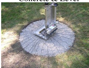
Radial Wires Installed Antenna Installed
